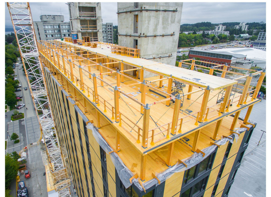
Acton Ostry Architects, Student Residence, Vancouver
