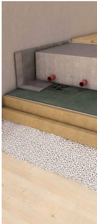
Fig. 3.47. Green waterproof membrane on top of the insulation (Rothoblaas, 2019).
