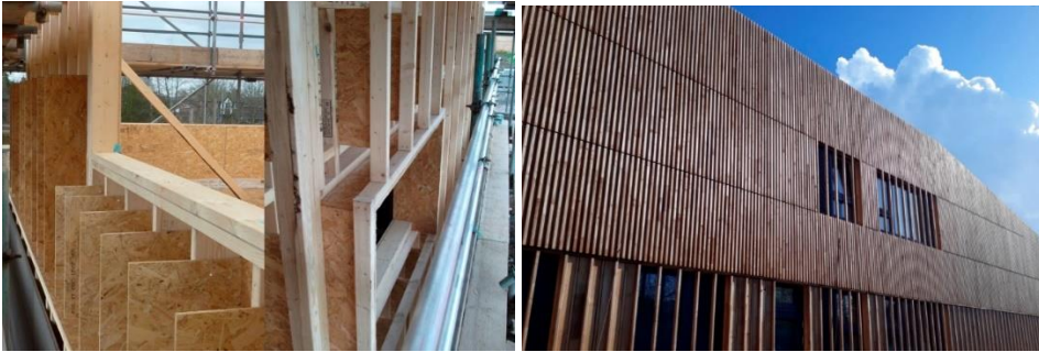
Fig. 1.37. Hackbridge primary school (Passivhaus Trust, 2020).
