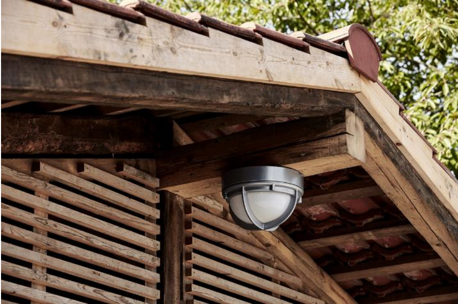
Fig. 7.40. Module facade (Photography Jonathan Weimar)
