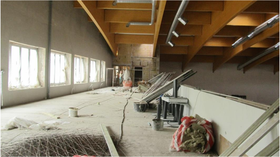
Fig. 7.21. The construction process of sports hall in Palanga city, Lithuania ( www.sporthall.palanga.lt )
