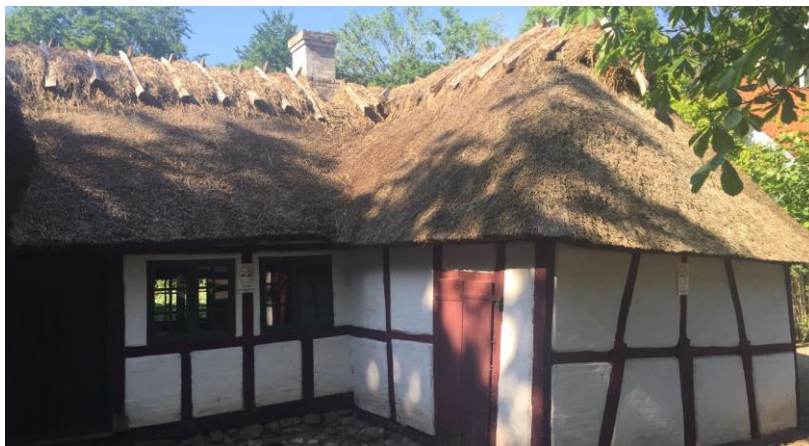
Fig. 3.13. Thatched roof in Denmark, Odense.
