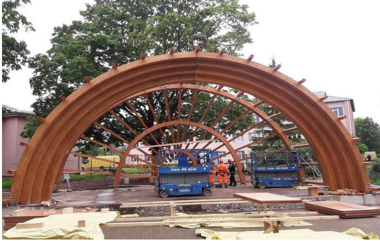
Fig. 7.4. Construction phase (GadalabākābūveLatvijā 2017, 2018; The best building of the year in Latvia, 2018)
