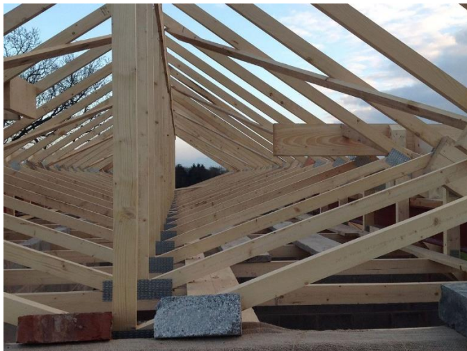
Fig. 6.39. Bracing of the roof (Minera, n.d.).
