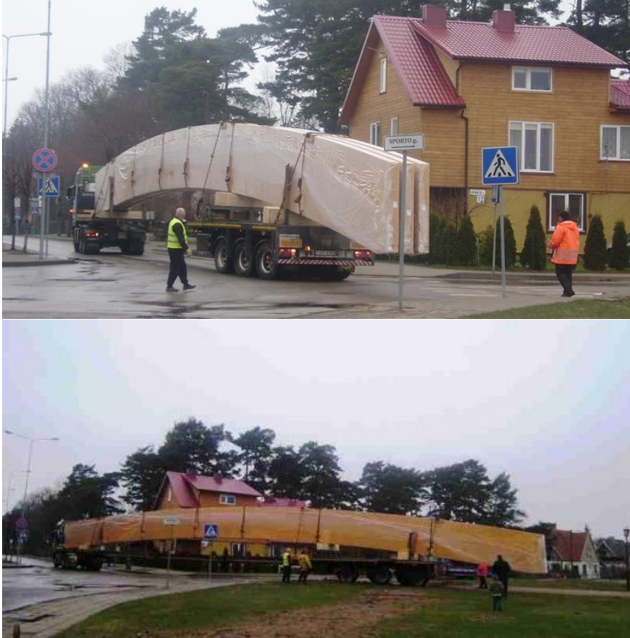
Fig. 7.20. The transportation of 36 m length glulam beams for the multifunctional sports hall in Palanga city, Lithuania ( www.veidas.lt )
