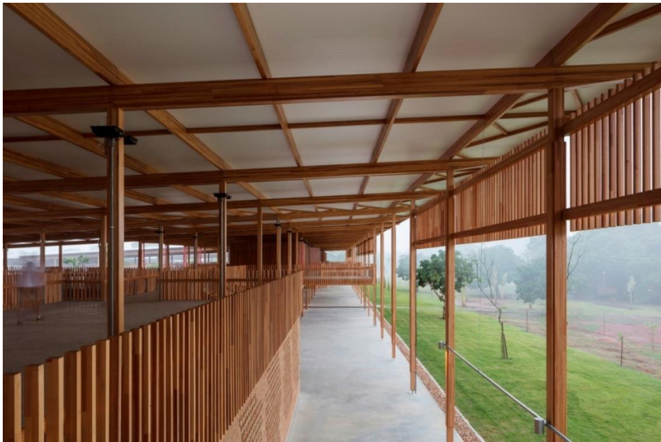
Fig. 7.54. Columns and roof structure (Leonardo Finotti - www.archdaily.com )
