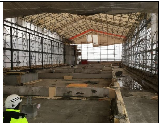
Additional floors construction, 7 th and 8 th floor, Tampere 2018.
