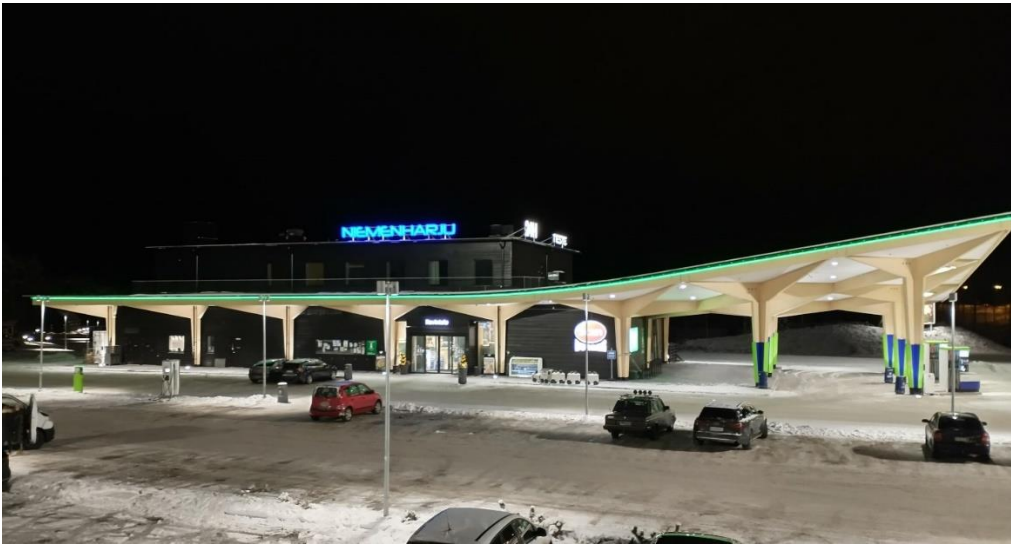
Fig. 4.4. The most beautiful fuel station of 2017. Glulam and CLT structure. 12/2020.
