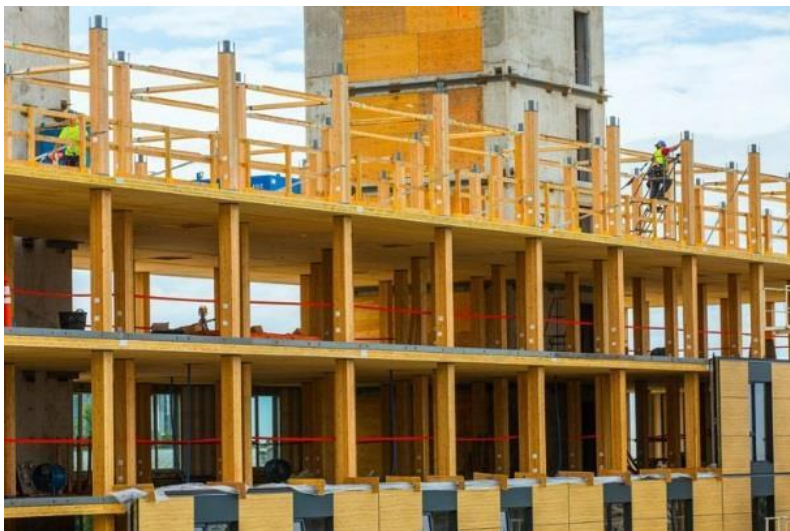
Fig. 1.10. Hybrid construction with glulam column and CLT beams. Source: Acron Ostry Architects, Photo: KK Law (cit. from InnoBYG, 2017).
