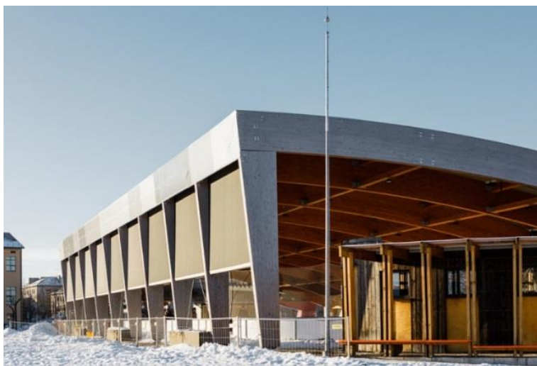
Fig. 7.12. Outside view (final view) (Gadalabākābūve Latvijā 2018, 2019. The best building of the year in Latvia, 2019).
