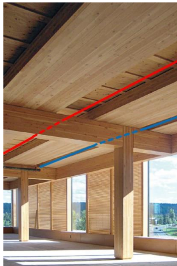
Fig. 3.41. Installations above the beams and between slabs.
