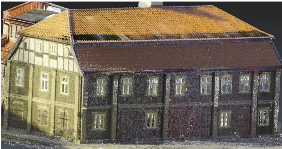
Fig. 6.1. Wood building in 3D point cloud after renovation (developed by authors).
