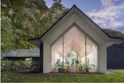
Fig. 7.26. The central hall ( www.e-architect.co.uk )
