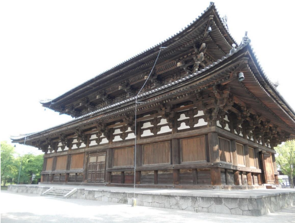
Fig. 2.20. Toji Buddhist Temple, Kyoto, Japan, dating from the 15 th century. © David Trujillo.
