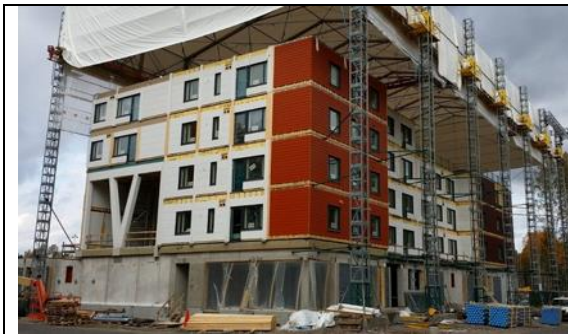
“The Gipson tower” is a steady rising weather shelter lift by motors. Assembly crane operates above the building under the shelter.
