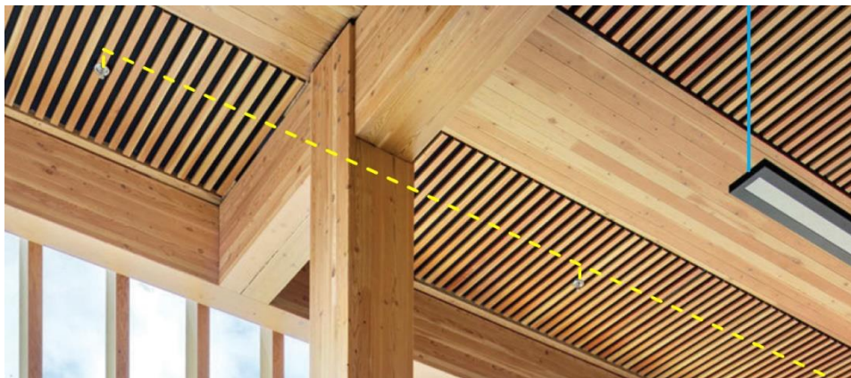
Fig. 3.42. Duct roads closed between the load-bearing CLT slabs.
