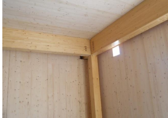
Fig. 2.18. Cross-laminated timber consists of orthogonally glued laminations. It is a versatile product that can be used as a slab or a wall, as seen here.
