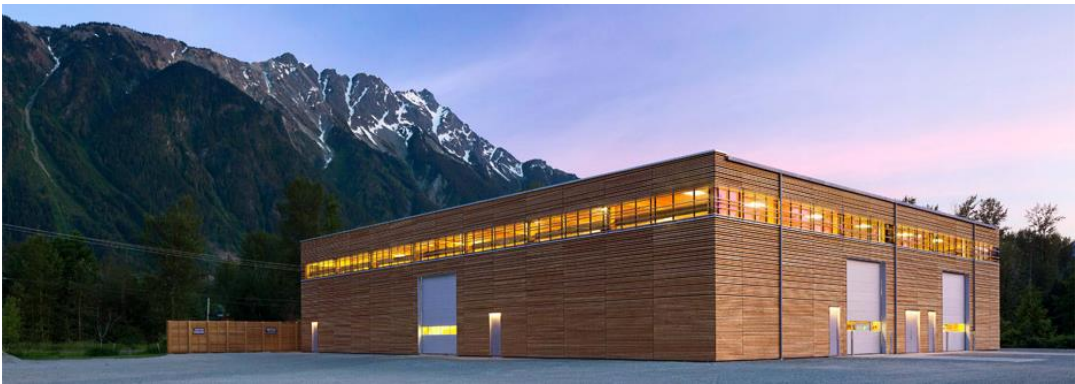
Fig. 1.40. The BC Passive House Factory (McKnight, 2016).
