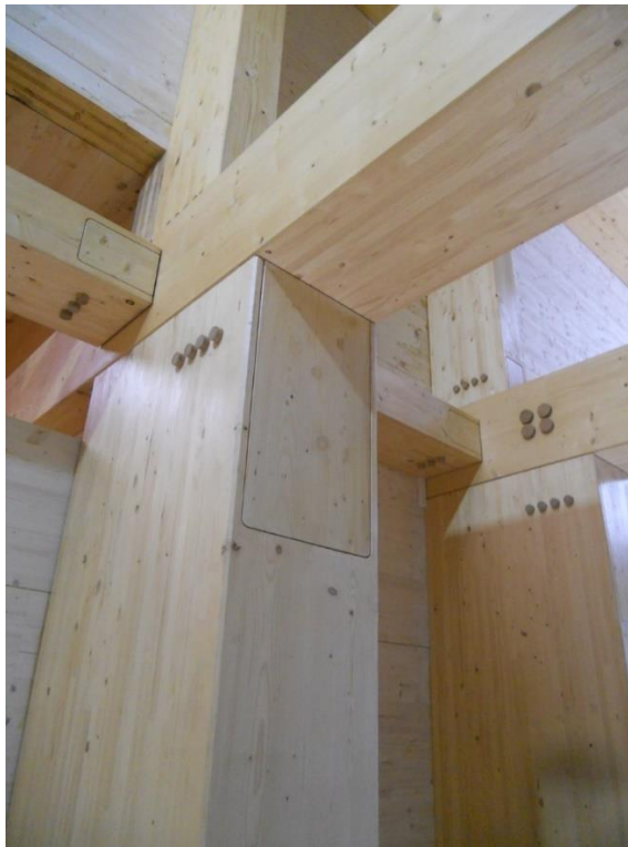
Fig. 2.28. Due to its better fire performance, timber conceals the steel beam-to-column connection – GlaxoSmithKline Carbon Neutral Laboratory for Sustainable Chemistry, University of Nottingham. © David Trujillo.
