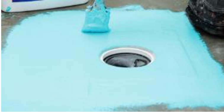
Fig. 3.12. Brushable water proofing in wet room
