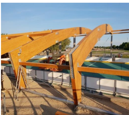
Fig. 7.15. Three-threaded frame (Gadalabākābūve Latvijā 2018, 2019. The best building of the year in Latvia, 2019).
