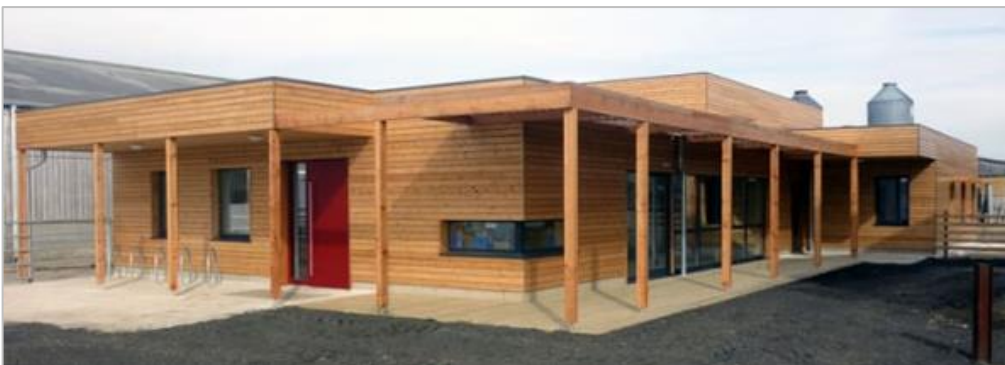
Fig. 1.39. Hadlow College (Passivhaus Trust, 2020).
