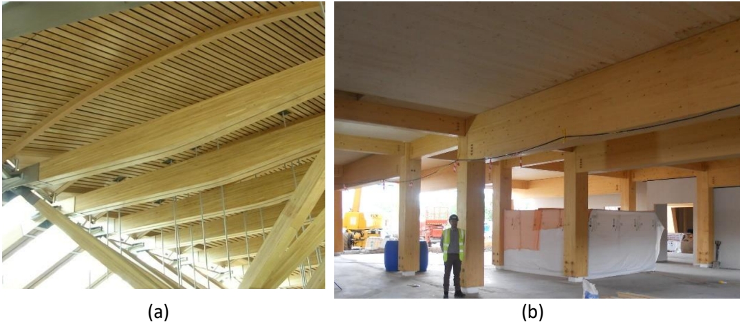
Fig. 2.26. Glued laminated timber, or glulam, is another engineered timber that can adopt varied shapes (a) and achieve very impressive sizes (b): (a) Scottish Parliament, (b) GlaxoSmithKline Carbon Neutral Laboratory for Sustainable Chemistry, University of Nottingham.
