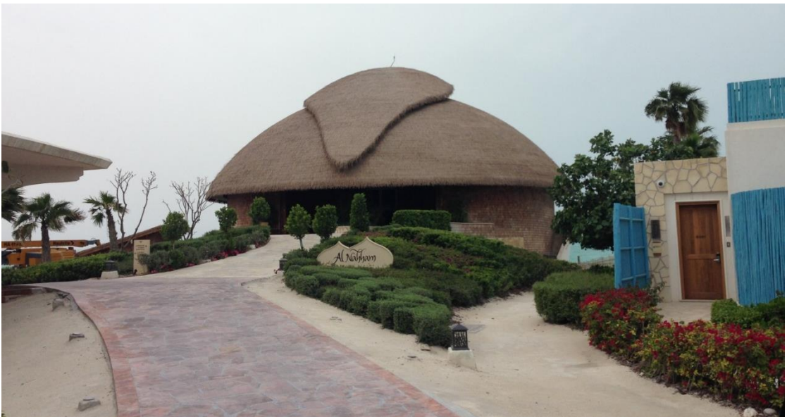
Fig. 7.55. The outside view of the lookout restaurant in Banana Island, Doha, Qatar
