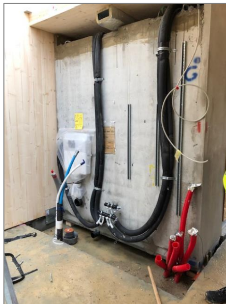
Fig. 3.53. Finished bathroom made of concrete (Byggeskadefonden, 2020).
