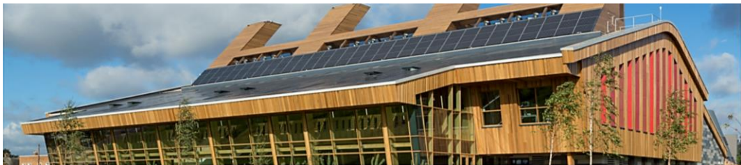
Fig. 1.25. GlaxoSmithKline, UK (BREEAM, 2020).
