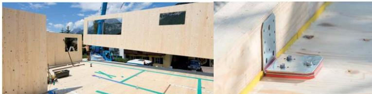
Figure 5: Elastic layers used for walls and connectors [4]
